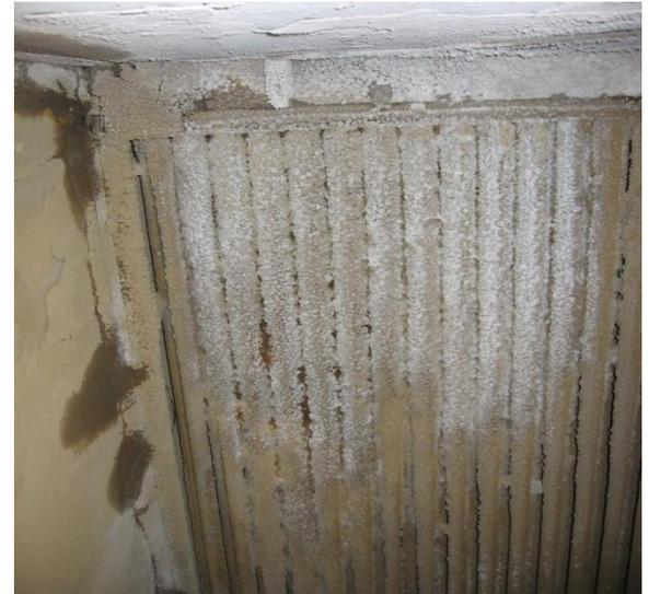
Watch<sup>®</sup> has noticed, the formation of process scale within heating and cooling equipment would not be noteworthy occurrence, except that these Heat exchangers are plugging on the water side instead of the process side of the tubes.
